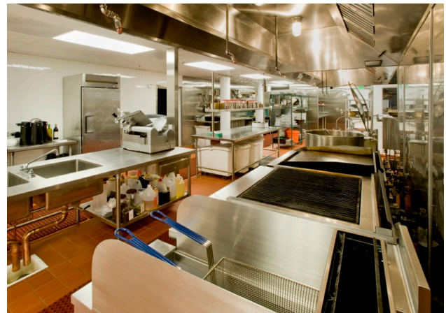
This photo illustrates the correct installation of a metal baffle plate between the open flames from the range and the deep fat fryer. Metal baffles should be used only when there is not sufficient space available to provide a 16" clearance between the deep fat fryer and any source of open flames. Baffle filters are seen above the range and fryer.
