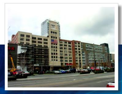
masonry) infill walls, which are known, in this day and age, to be prone to failure when faced with an earthquake or high wind pressure. Fortunately, about a year before the earthquake, the building had been seismically retrofitted.
